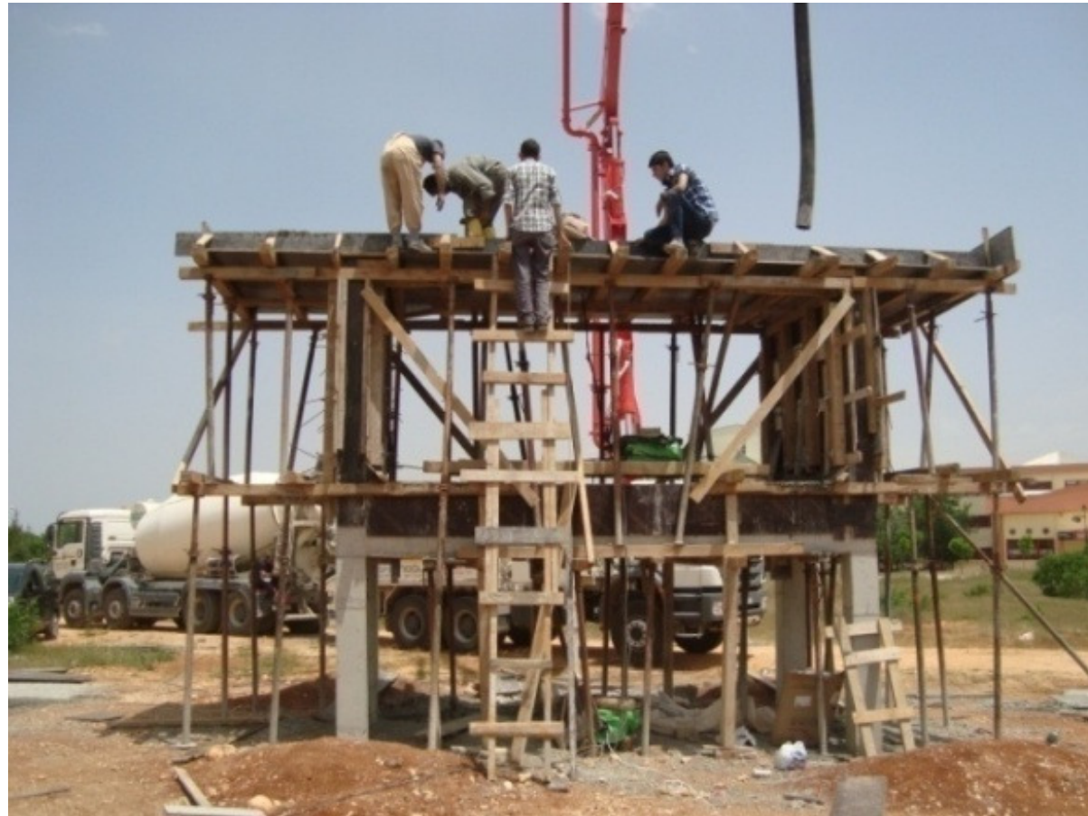
Figure 1: Concrete casting of the experimental full-scale box-girder segment
