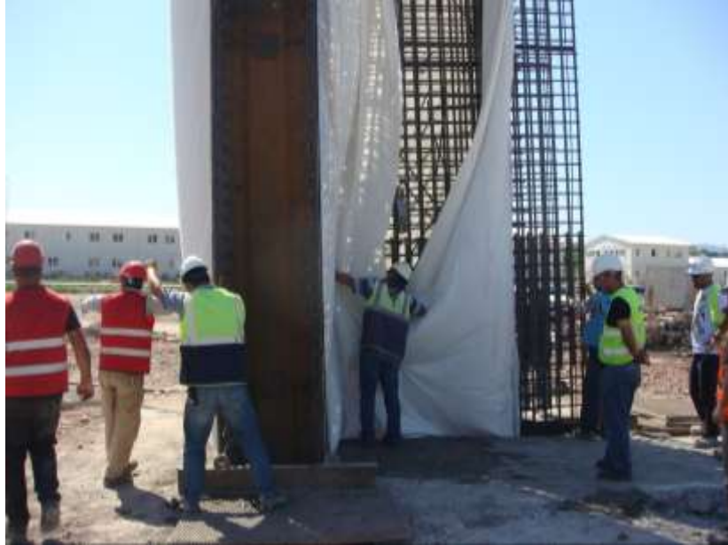
Figure 10. Covering the reinforcement cage with geotextile
