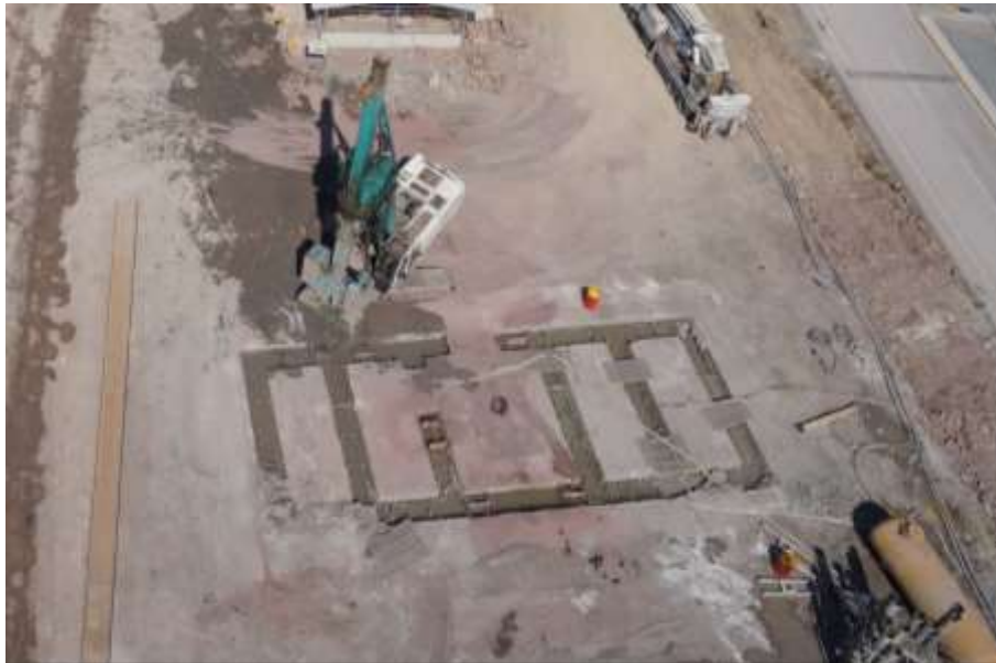
Figure 7. Diaphragm Wall Panel Excavation
