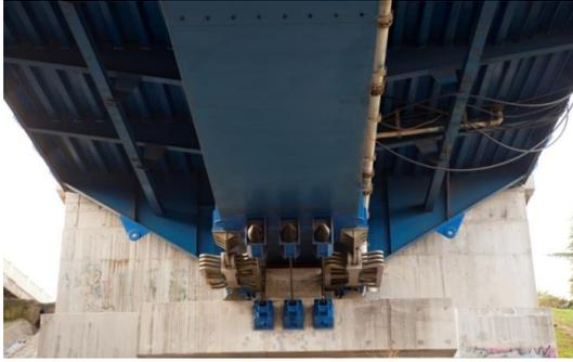
Figure 5. Damper and falling down prevention jacking at Golden Horne Bridge.
