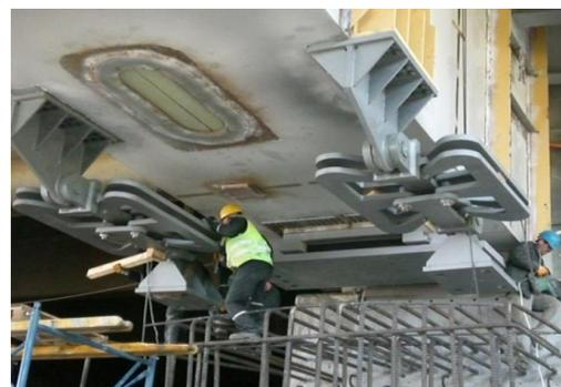
Figure 4. First Bosphorus Bridge damper installation.
