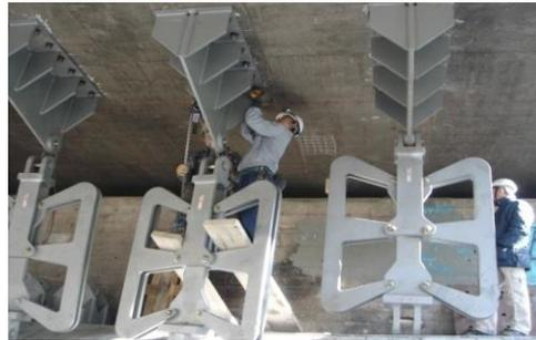
Figure 9. Damper installation at Old Golden Horn approach viaduct abutment.
