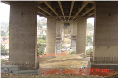
Figure 8. Retrofitting of piers with concrete jacking at Ortaköy V408 viaduct.
