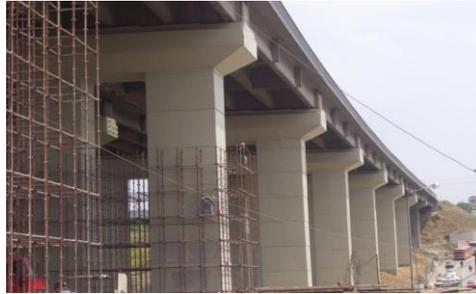
Figure 12. Retrofitting of piers with concrete jacketing at Sagmalcilar viaduct.
