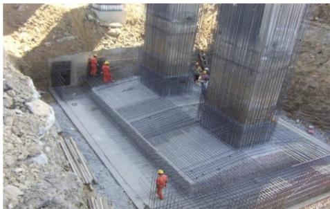
Figure 10. Retrofitting of footing at Mahmutbey viaduct.
