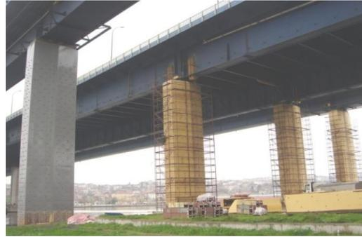
Figure 6. Retrofitting of piers with steel jacking at Golden Horne Bridge.
