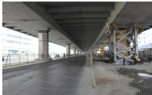
Figure 11. Installation of LRB bearings and retrofitting of piers with steel jacking at Mecidiyeköy Viaduct.
