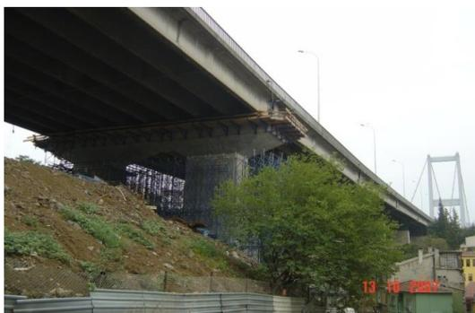
Figure 3. Retrofitting of cap beams at Bosphorus Bridge approach viaducts.
