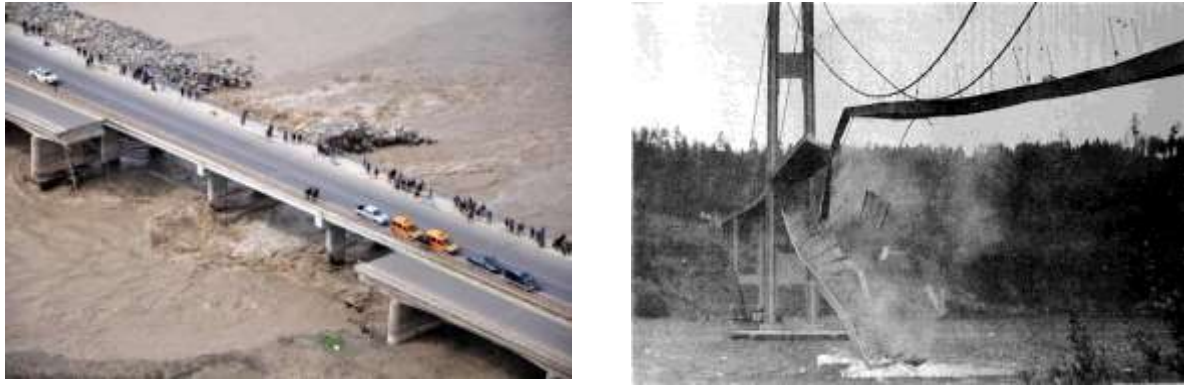
Figure 1. Two examples of disastrous bridge collapses. Right-Çaycuma, Turkey, 2012. Left-Tacoma Narrows Bridge, 1940.
