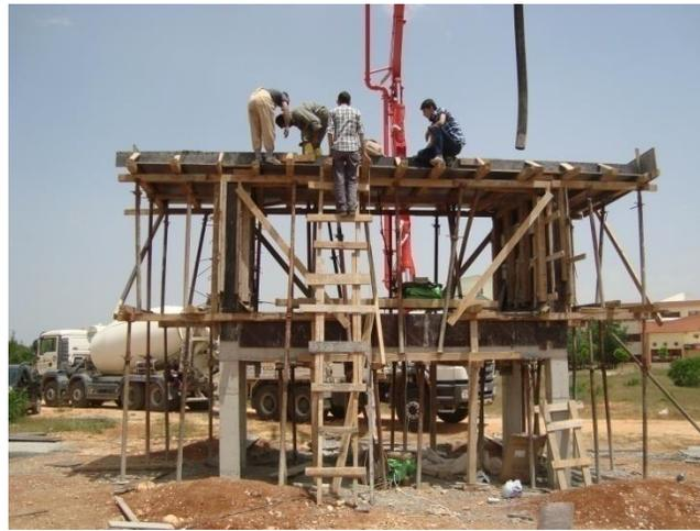
Figure 2 Concrete casting of the experimental full-scale box-girder segment
