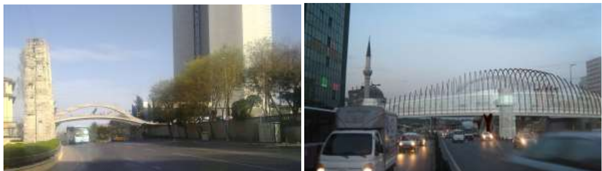
Fig. 4, Yeni Gezi footbridge; Fig. 5, Şirinevler footbridge
