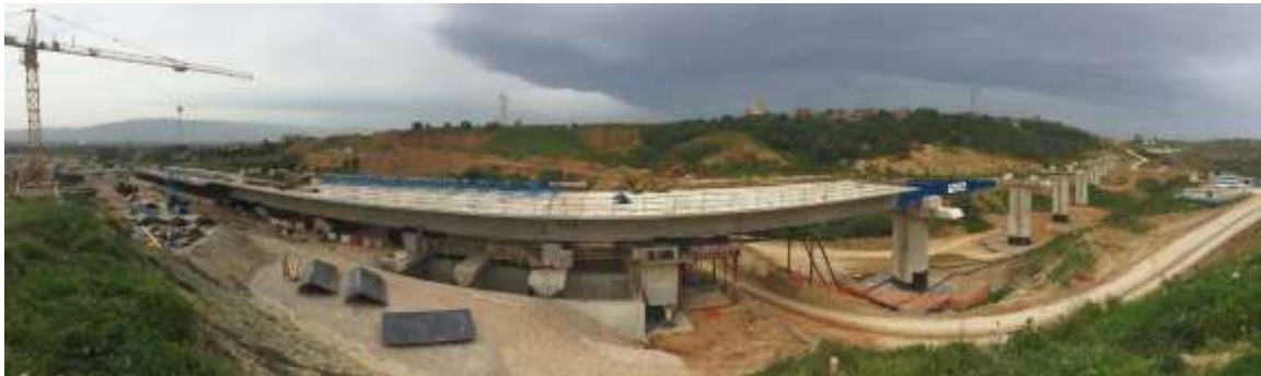
Figure 7. BTZ Bridge in movement.
