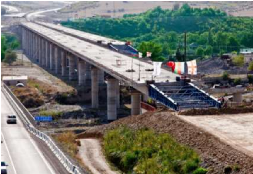
Figure 10. Liakhvi Viaduct close to completion.
