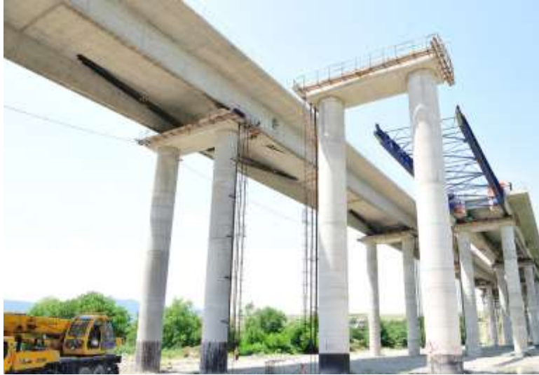
Figure 9. Liakhvi Viaduct during launching.
