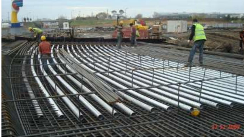
Figure 15. Curved tendon ducts being installed (Ataturk Airport-Istanbul).
