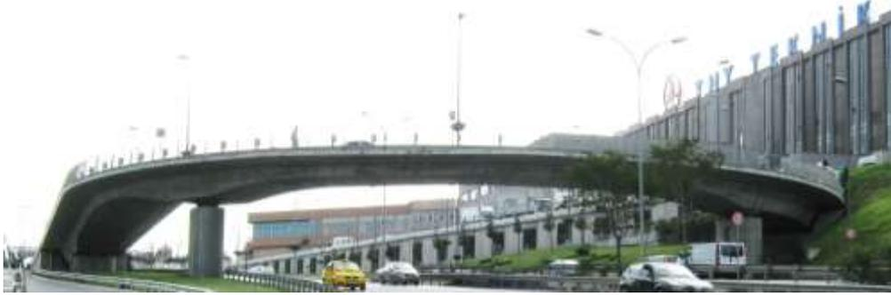
Figure 5. Continuous post-tensioned variable–depth curved bridge at Ataturk Airport.
