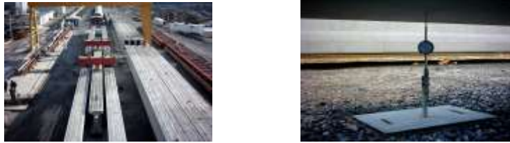
Figure 14, 15. Applying load over beams and deflection measurement.
