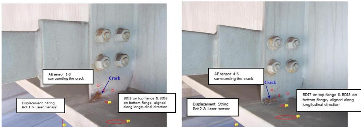
Figure 3. Crack at G3B2D3 (Girder 3 Bay 2 Diaphragm 3, left) and G4B3D3 (Girder 4 Bay 3 Diaphragm 3, right) and sensor locations.
