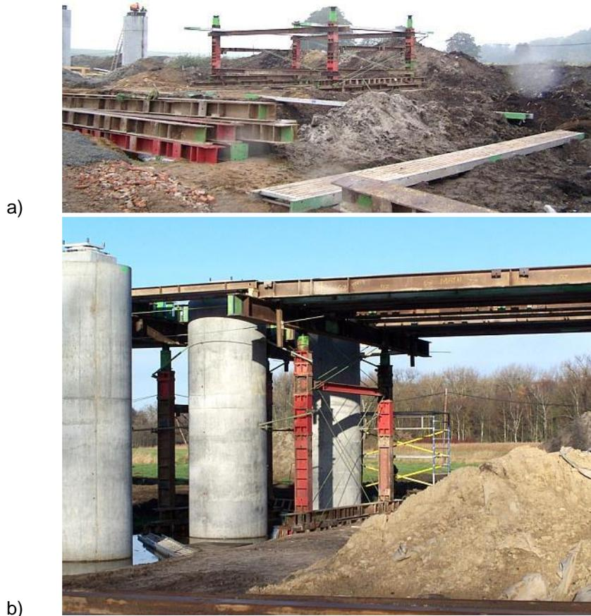
Figure 9. Construction of falsework supports: a) at midspan – two braced frames, b) near viaduct pier – a simple frame internally braced.
