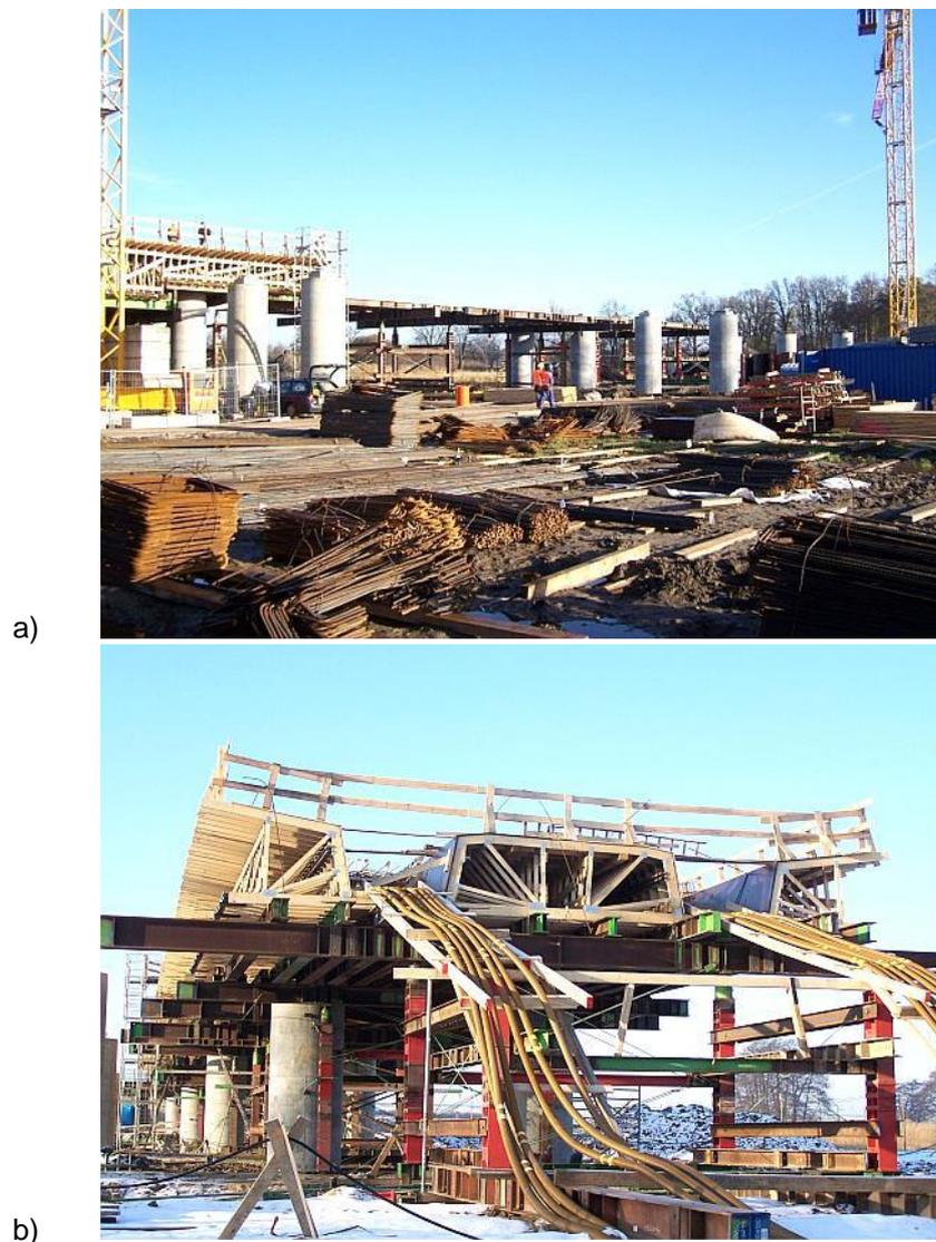
Figure 12. Falsework for the next stages of the north deck construction: a) general view, b) front view, after timber panel assembly and placement of reinforcement and cables.
