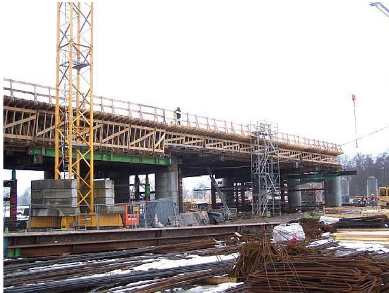
Figure 13. General view after falsework transversal movement and assembly of timber panels for the south deck: stages 1 and 3.
