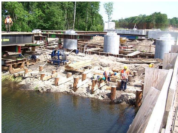
Figure 14. Last stages of construction: assembly of steel beams for the north deck and timber piling for the south deck, on the left – the temporary bridge.
