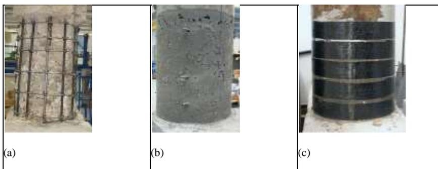
Figure 1 Proposed rapid repair and seismic retrofitting solution for damaged Italian pier: a) damaged rebar part substitution, b) concrete restoration and c) seismic retrofitting by C-FRP wrapping.
