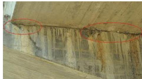
Figure.8 Tight contact between slab bottom and bent cap
