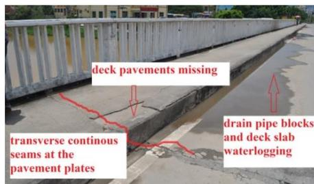
Figure.9. Rupture of bridge deck and side walk pavement
