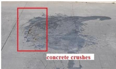
Figure.7 Pavement concrete crushing
