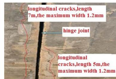
Figure. 4. Cracks on the bottom of beam
