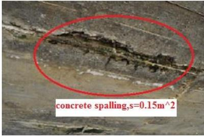
Figure.5. Concrete spalling
