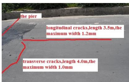
Figure.3. Cracks on the top of bridge deck
