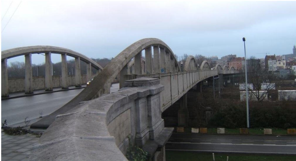
Figure 2. Rampe du Lion bridge crossing railway tracks at Schaerbeek
