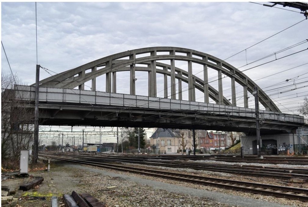
Figure 3. Bridge Dendermonde crossing various railway tracks
