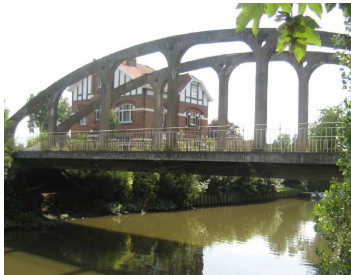
Figure 1. Pontweg bridge across river Lys
