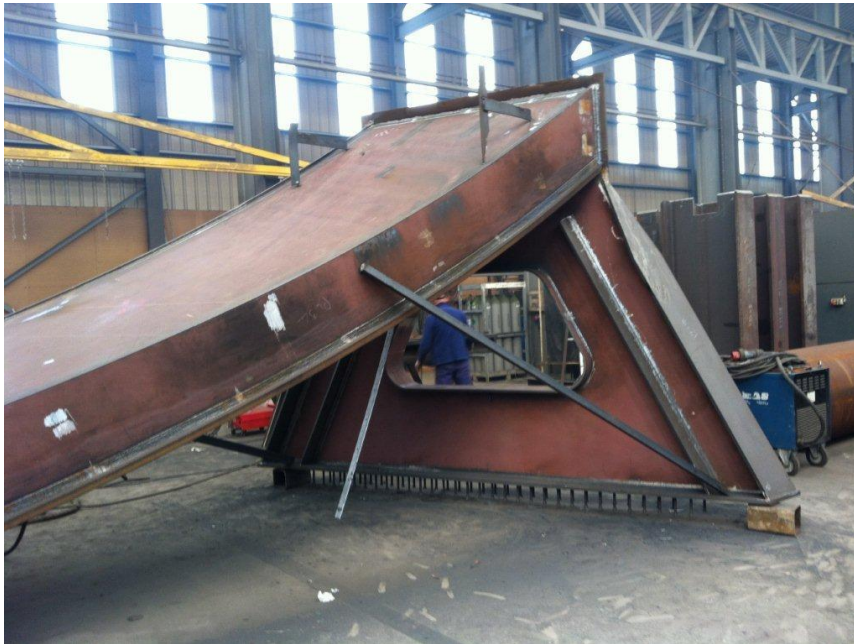
Figure 4. Assembling of arch box section to diaphragm stiffening strut
