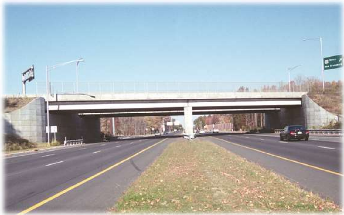
Picture 1. T-WALL Abutment
