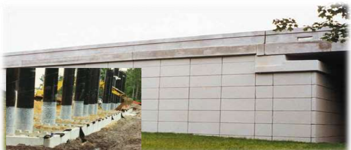
Picture 2. Pile Supported Bridge with T-WALL Abutment
