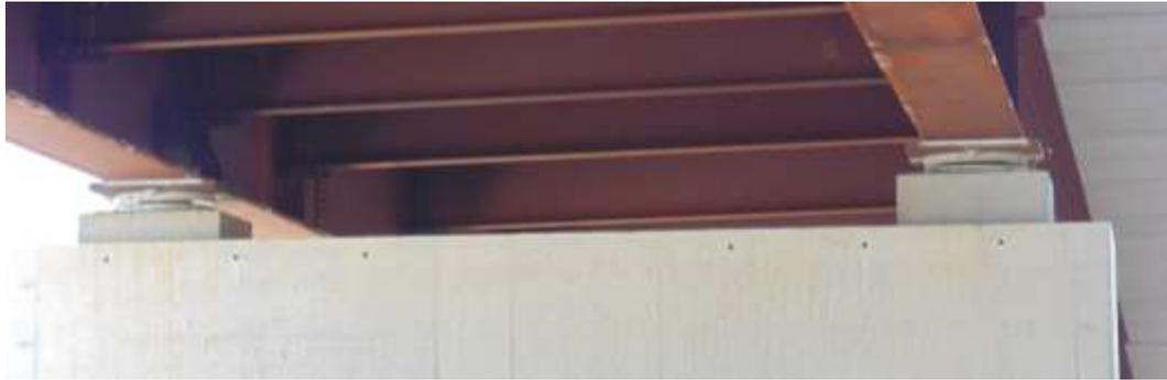
Figure 18. Casale Civile viaduct. Deck intrados on new pendulum isolators.
