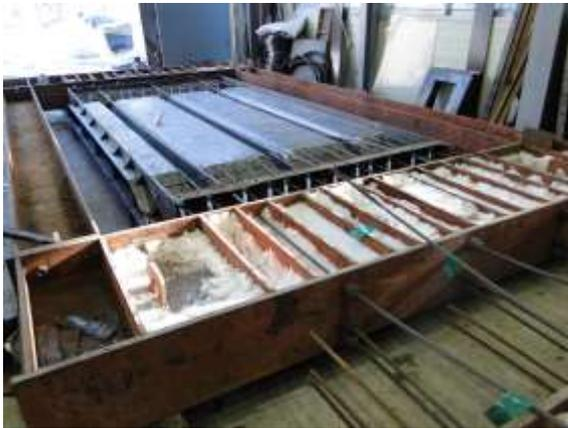
(a) Assembly of form and arrangement of reinforcement
