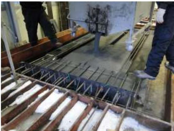
(c) Placing of UHPC of precast part
