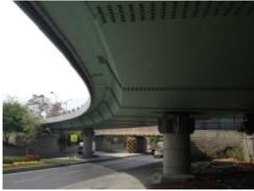
Figure 1.1. General view of the bridge.
