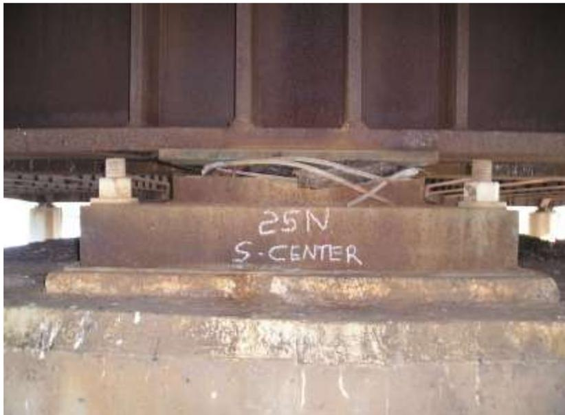
Figure 2. Pot bearing with sealing ring failure.
