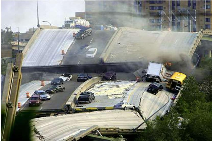
Figure 6. Collapse of the I-35W bridge in minneapolis.
