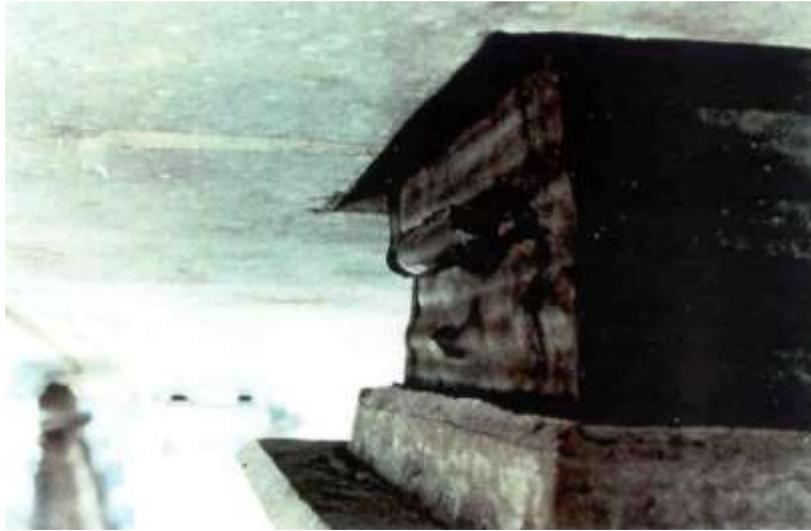
Figure 1. Elastomeric bearing pad exhibiting excessive deflection.
