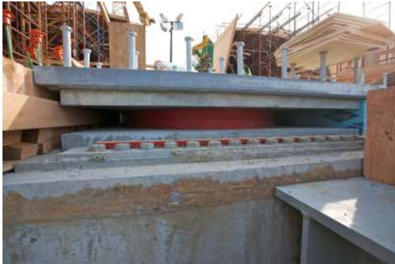
Figure 10. HL MDB installed on I-35W bridge showing containment plate.
