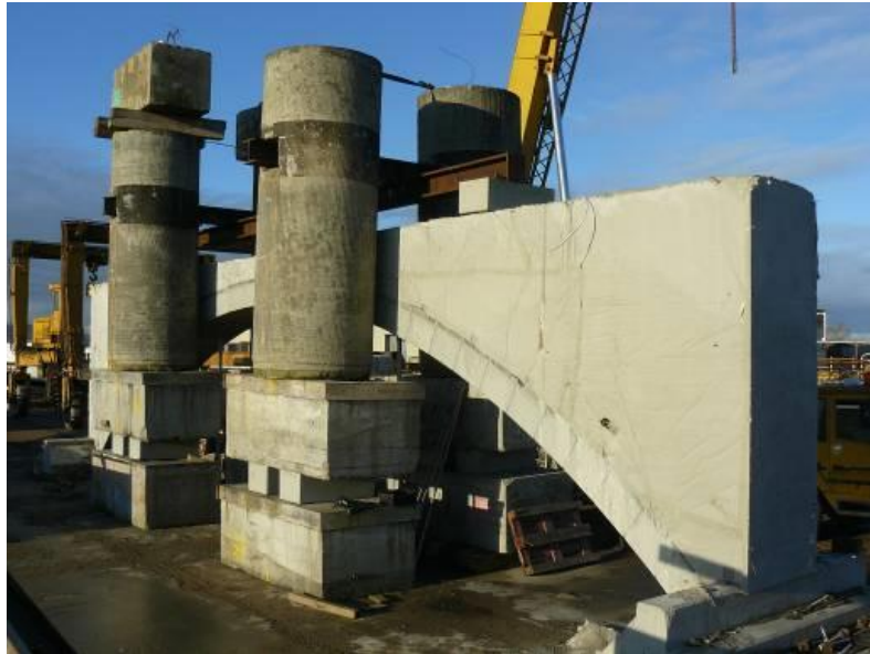
Figure 2 Testing full scale 15m span x 3m rise FlexiArch
