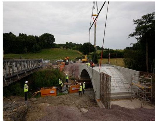
(b) Nearing completion
