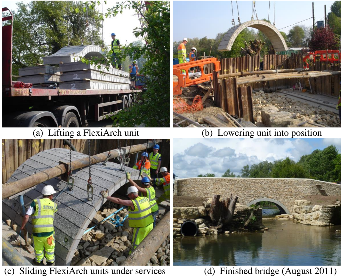
Figure 5 Siddington, UK- avoiding disruption to services
