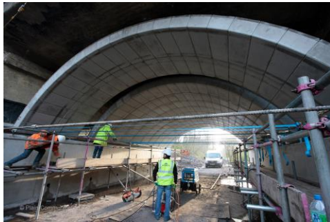
(c) Sliding FlexiArch units along sill beams
