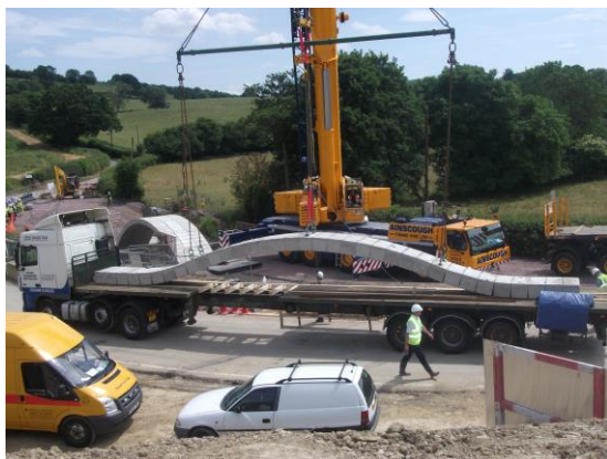
(a) Lifting 13t FlexiArch unit
