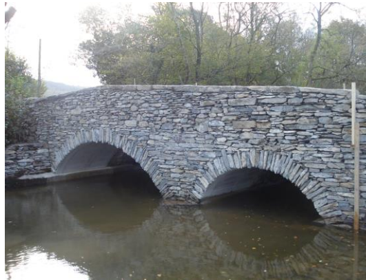
(c) Finished bridge (October 2011)
