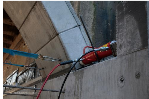
(b) Hydraulic jacking system
