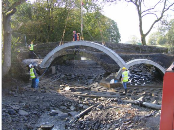
(a) Lowering longer span unit onto sill beams
