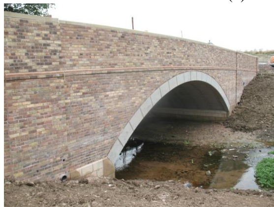
(c) Finished bridge (October 2010)
