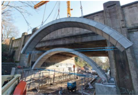
(a) Installing FlexiArch unit on extended sill beams utilised
