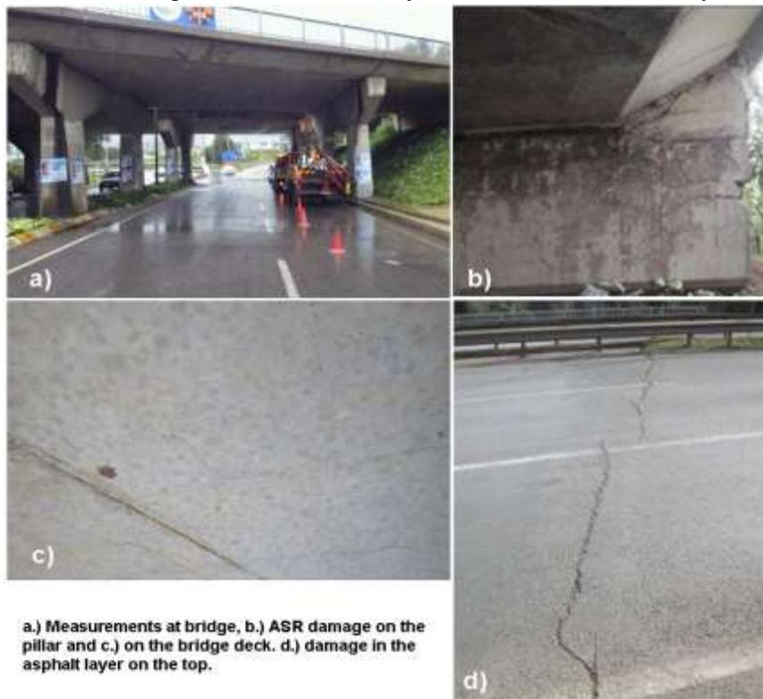
a.) Measurements at bridge, b.) ASR damage on the pillar and c.) on the bridge deck. d.) damage in the asphalt layer on the top.
