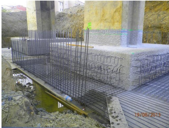
Figure 10: Retrofitting of Foundations
