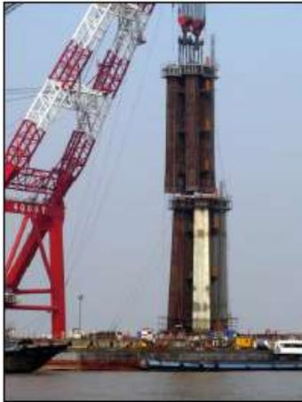
Figure 9. Tower tier trial fit-up
