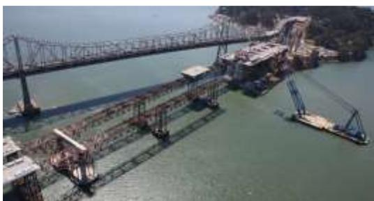
Figure 6. Temporary truss falsework
