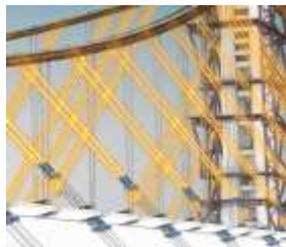
The key issue for the erection of the SAS was the load transfer of the box girders from the temporary trusses to the cable system. This took place after the box girder had been assembled on the trusses, the main cable was erected and compacted, the cable bands bolted in place, and the hangers hung from the cable. The load transfer was accomplished by progressive jacking of the hangers until they could be socketed to the box girders (Fig. 15).
